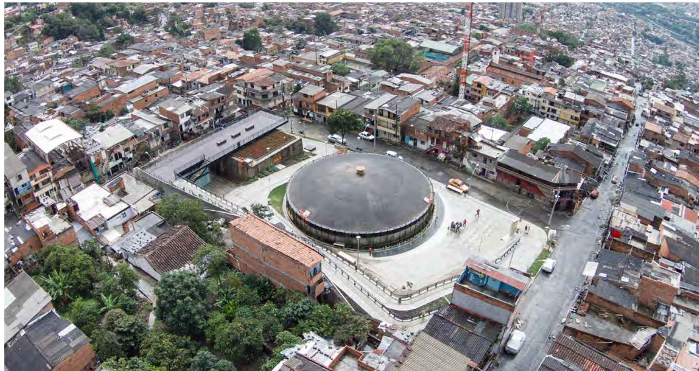
Original Infrastructure: Moscú Tank Neighborhood/Commune: San Pablo, Popular Design and Construction: January 2013 - March 2014
