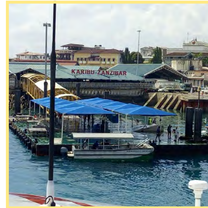
1- Zanzibar ferry terminal
